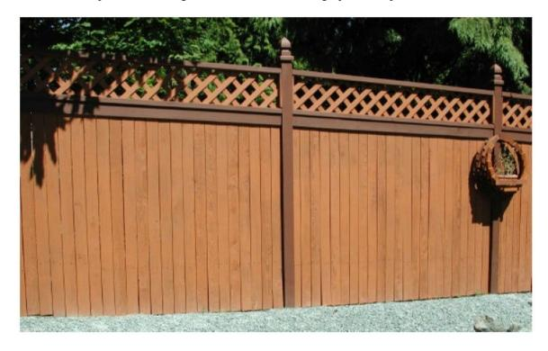
The fence design adopted and approved by the Board is shown here. It is 72" tall, constructed from 1 x 4 cedar with a 12" cedar lattice strip across the top. Support posts need not be cedar, but can be pressure treated lumber.
